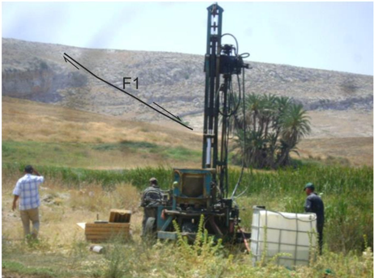
Figure 3) A geotechnical survey by rig with the presence of a fault F1 with traces on of Eocene age and embedded in the Reservoir.
